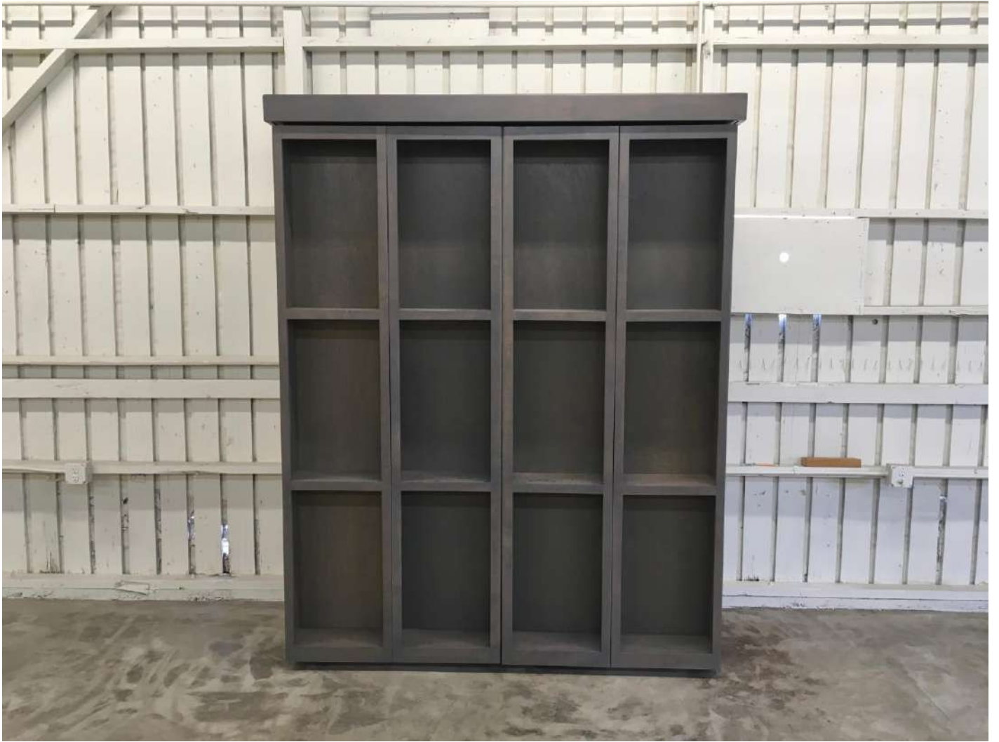
(Finished) THIS IS THE RESULT OF THE INSTALLATION.
