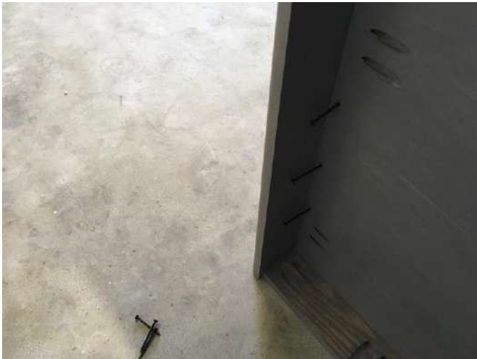
(7) Once both side and frame line up, then screw in the top with the 2 ¼" drywall screws supplied.
