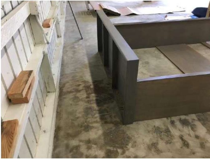
(5) Using the 2 ¼" drywall screws supplied, you can begin by installing the top piece to the overall unit.
