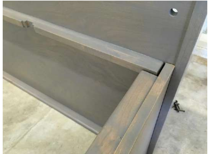
(6) There's 2 aspects of installing the top piece that are very important:
